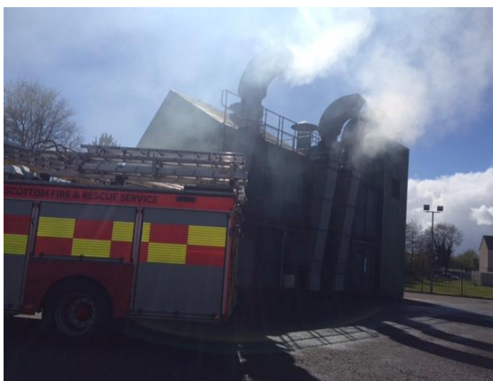
Falkirk Fire Station, 40 min unna Hq.
